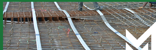
SLAB & SPIRAL DUCT
