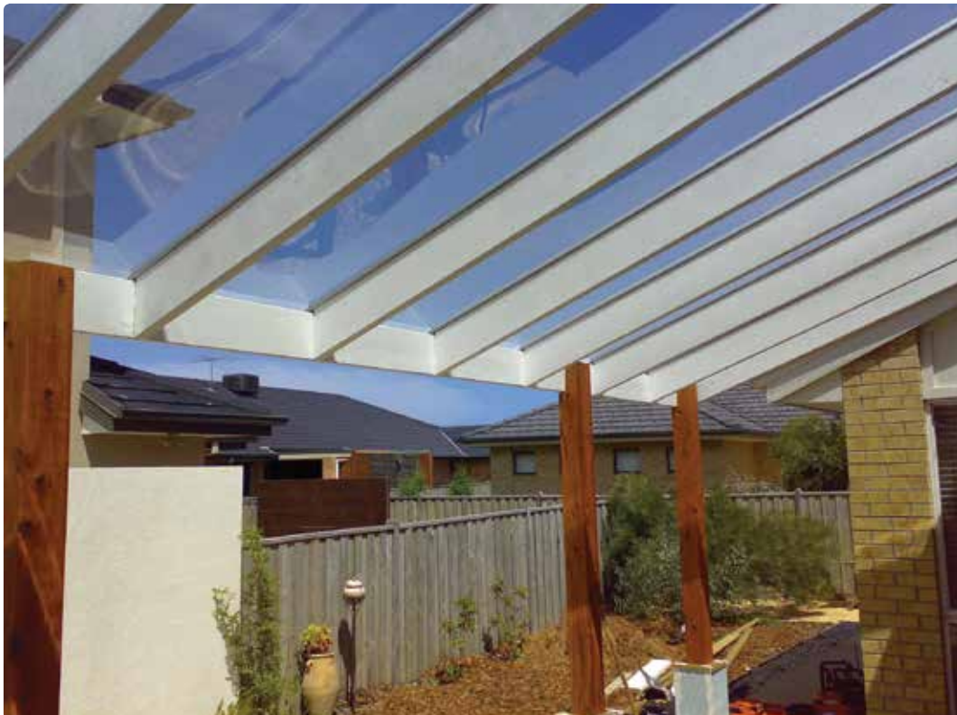
Project: Private home, Point Cook, Australia | Application: Pergola | SUNGLAZE™ Type: Clear 4mm
