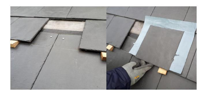
Step 4: Snap the piece into place <u>without removing the protective film</u> (otherwise you won't be able) and once the membrane is below the edge of the upper row, remove the film.
