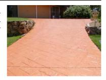
**General Application Guide:** Apply one coat of Shieldseal X clear primer by nap roller as a primer coat. Allow to dry for 24 hrs.
