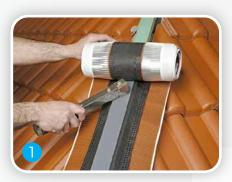
A UV stabilized fleece is placed over the ridge, with up to 50% stretch for ease of installation and butyl strips for adhesion. Using an advanced labyrinth technology, the fire resistant fleece allows air to be released but keeps the roof ridge weather tight (tested by CSIRO Aus/NZ 404.9 'Dynamic Weather Resistance').
