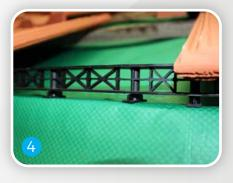
The Eaves Comb filler sits on the eaves board under the last course of tiles and allows the air to continually circulate up under the tiles. This continuous circulating air prevents heat from the tiles radiating through the roof.
