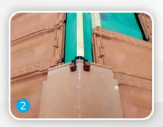
The ridge clips have been designed especially for the Australian market to fit the most common roof tile profiles. Each ridge cap is held securely in place with the clip. The ridge caps are fixed securely with the clips to the ridge batten.
